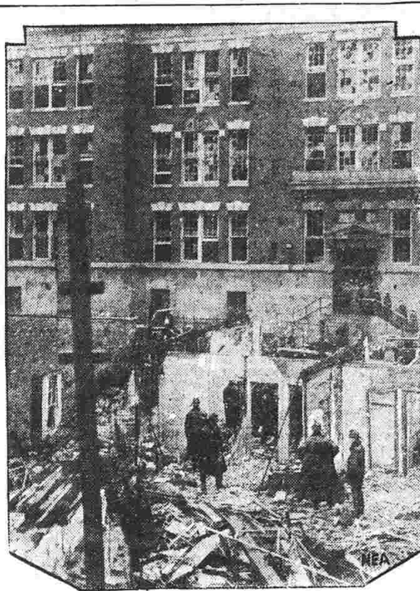
Like a scene on a war-torn battle front is the one pictured here after an explosion of accumulated gas had wrecked a house in Brooklyn, N. Y., and rocked the school building shown in the background, injuring more than 20 pupils, many of whom were taken to hospitals. Here you see how roofs and walls of the dwelling were shattered by the terrific blast. Two thousand pupils were attending classes when the explosion occurred.
